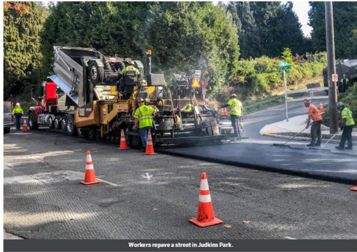
Workers repave a street in Judkins Park.
